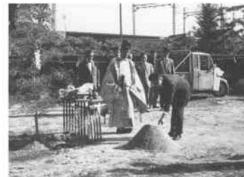
Shinto ceremony of purifying a site for new head office building (completed on June 2, 1963; 31 years old)
